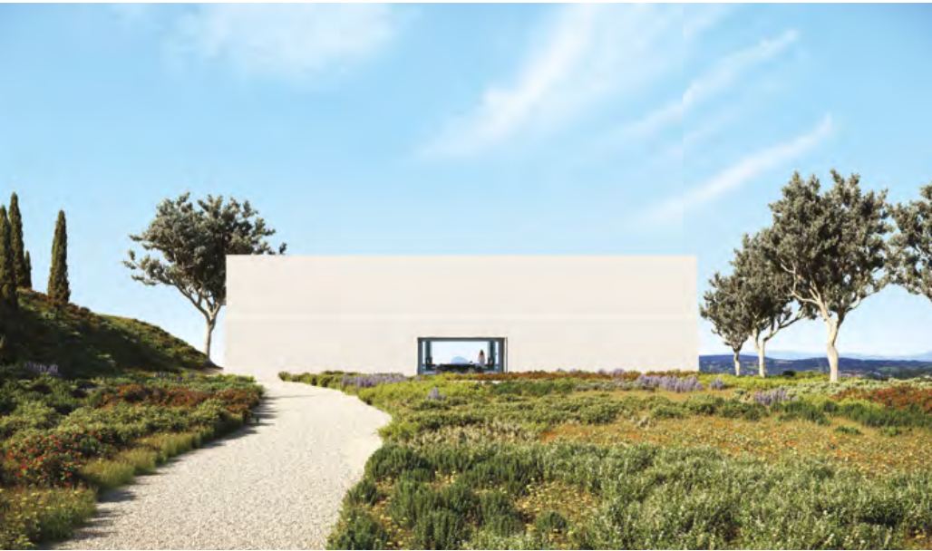
The approach to one of The Seven designed by Andreas Martin-Lof Arkitekter, Stockholm
