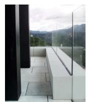
Glass parapets fixed to the slab or masonry using steel profiles, neoprene base pads, and black silicone sealant.
